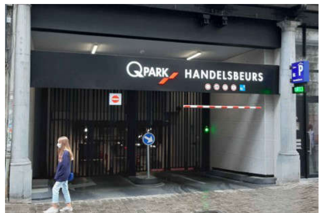
Name indication facade
