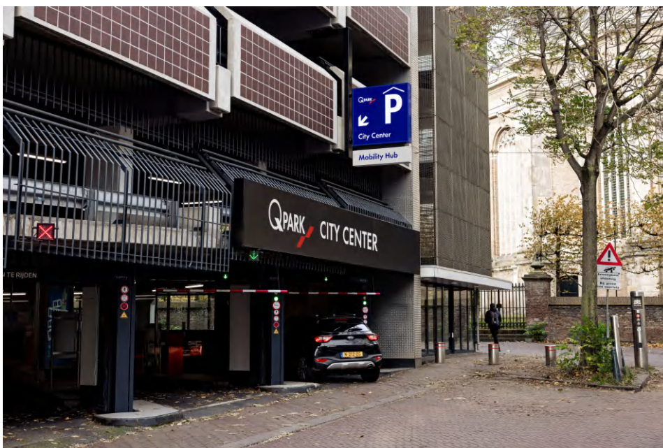
P-sign perpendicular to the facade
