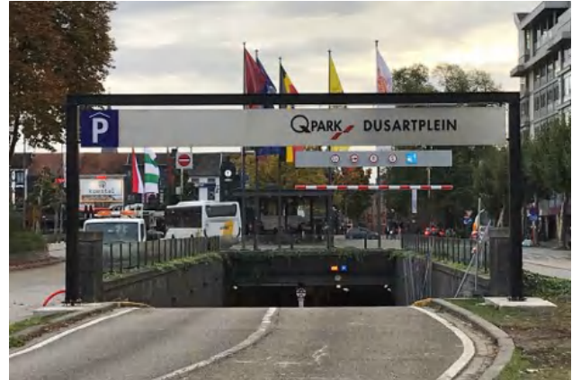
Entrance portal U-shape
